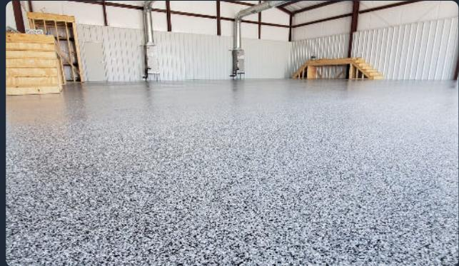
Epoxy flake flooring combines exceptional durability with an attractive, textured appearance. Vinyl flakes are broadcast into the epoxy layer, creating a speckled finish that conceals minor imperfections while providing excellent slip resistance.
